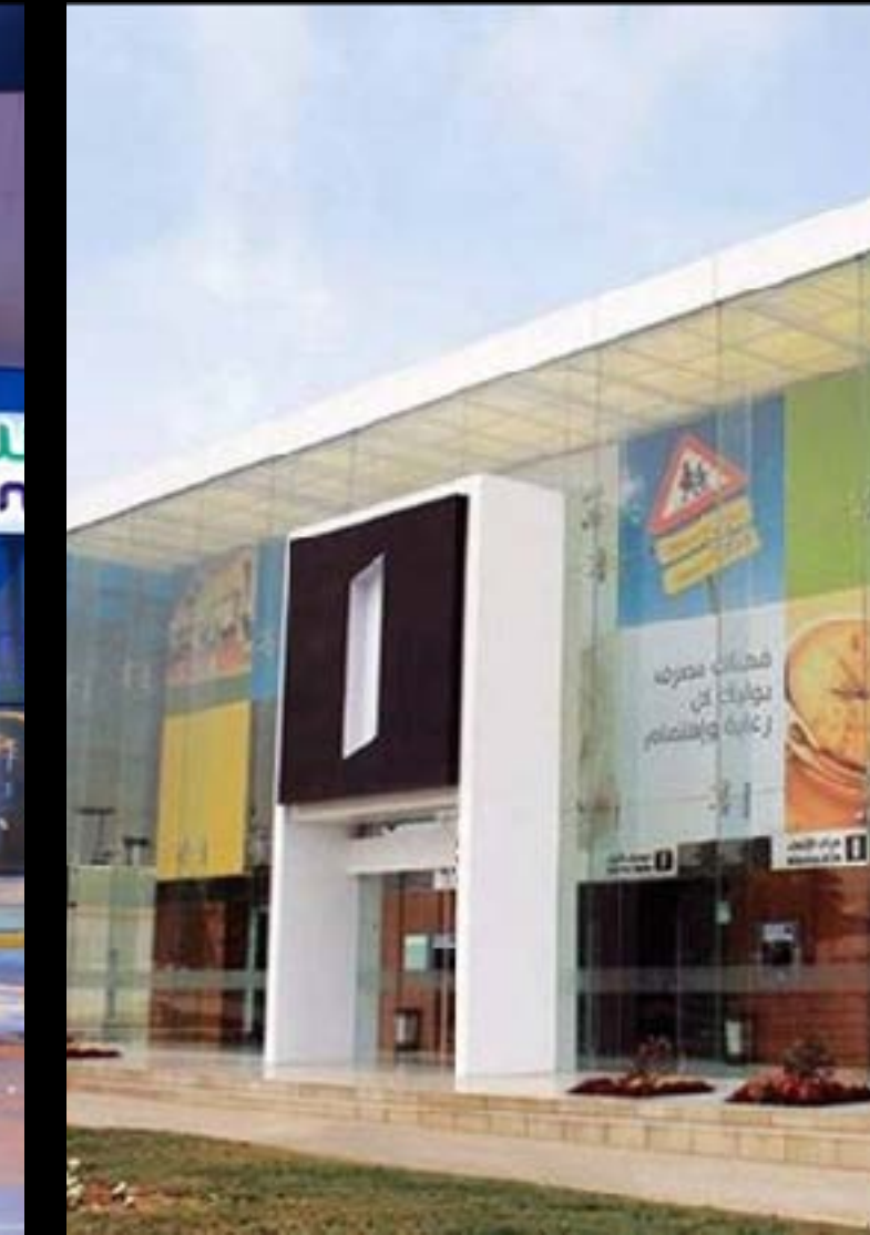
ALINMA BANK BRANCHES MULTIPLE CONTRACTORS
