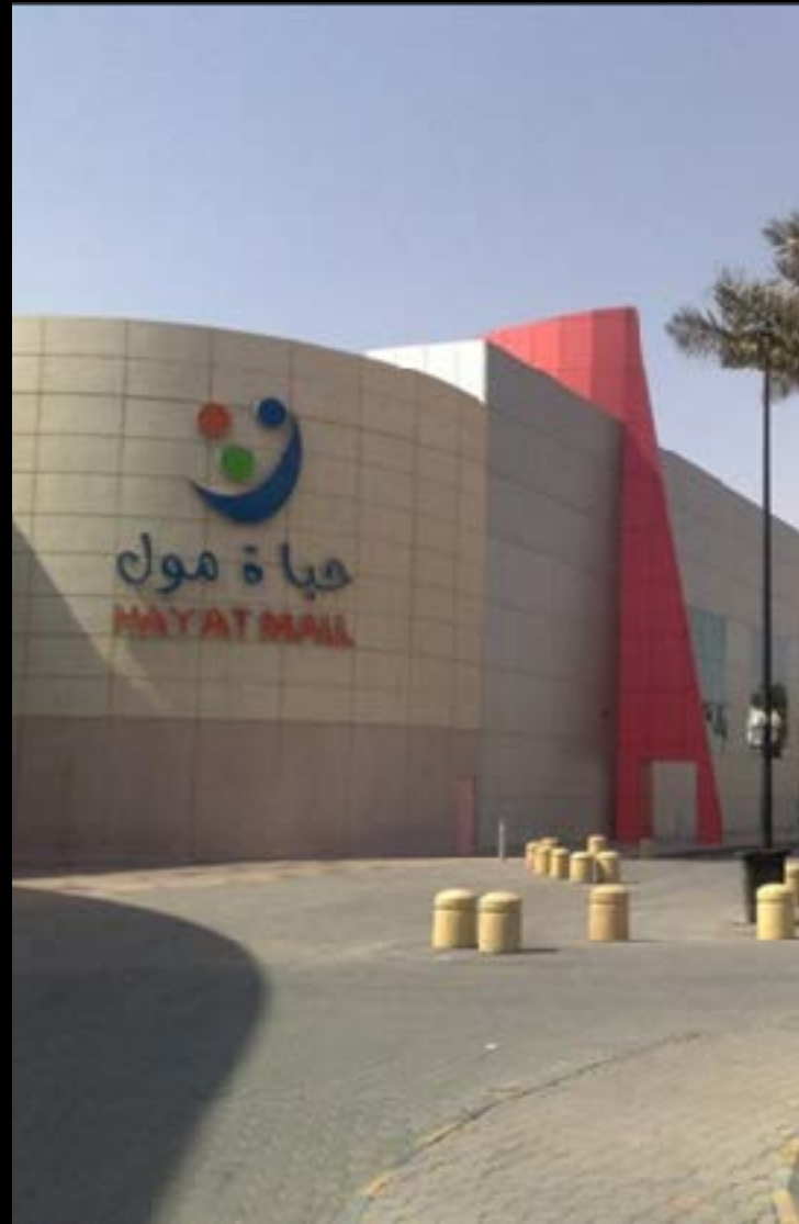
HAYAT MALL EXPANSION PROJECT
